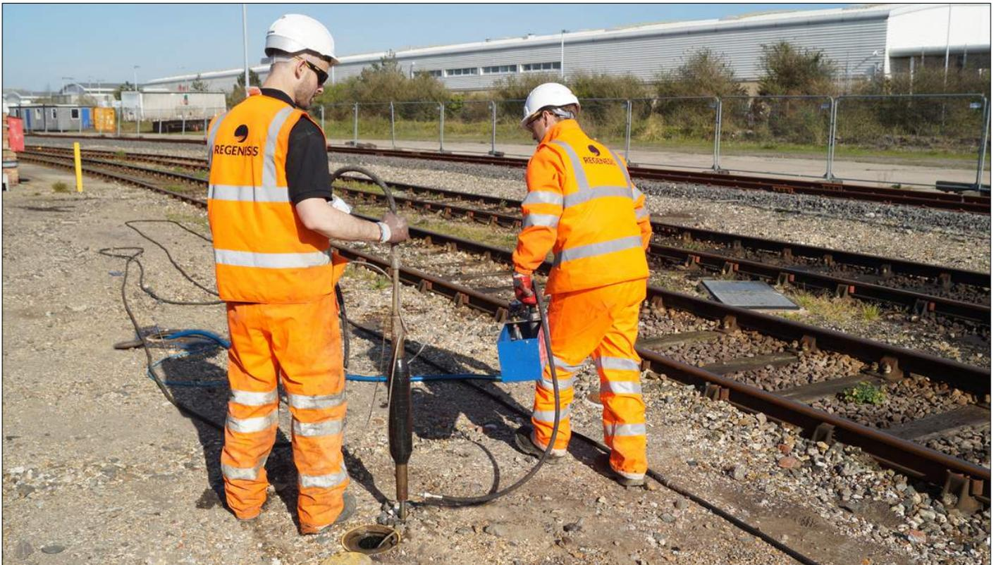
The first phase comprised the installation of a pump and treat (P&T) system enhanced with PetroCleanze in order to rapidly remove the LNAPL and adsorbed contamination in the smear zone. 18 treatment wells and 10 monitoring wells were installed across the target area: along the access road, the fuel point and within the four foot and six foot of the rail.
